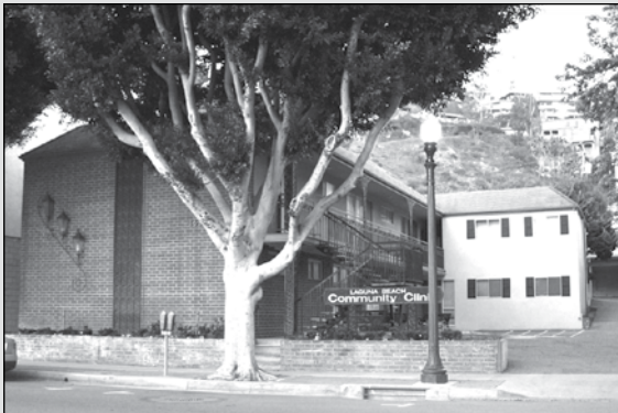
The new face of the Clinic with fresh landscaping & paint
